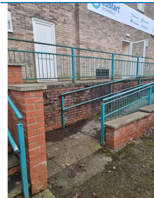
Access ramp with handrails to the main building entrance.
