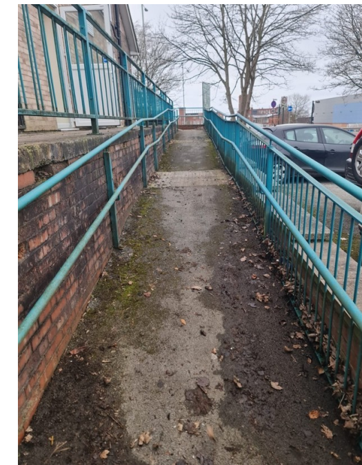
Ramped, railed walkway providing a step-free route to the site.
