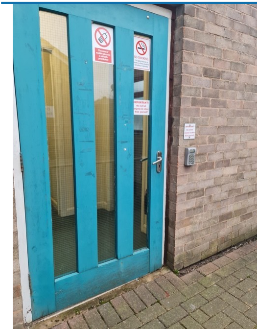
Side door fitted with a keypad/intercom entry system.
